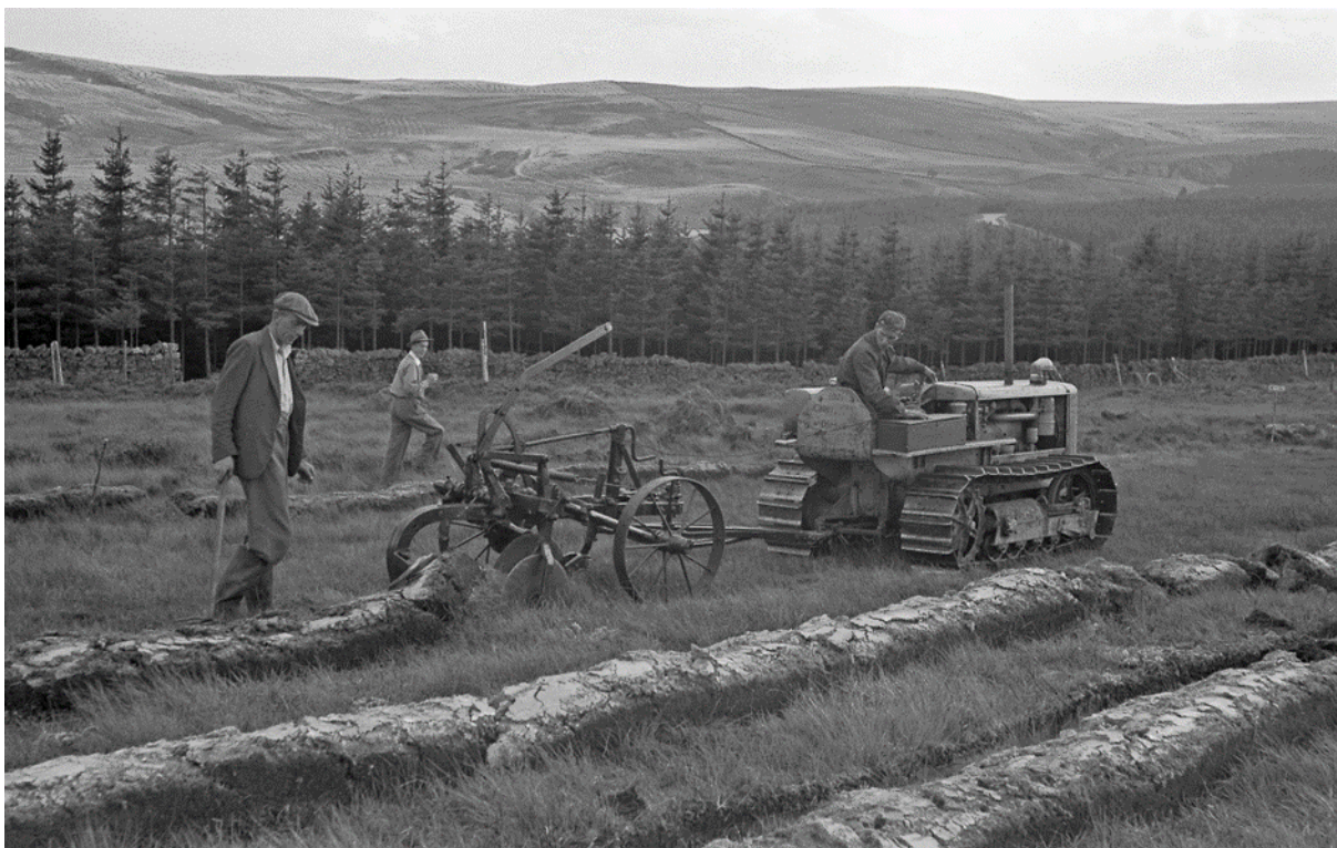
Figure 3. Early plough and D2 Caterpillar Tractor, 1946. © Crown Copyright Forestry Commission, Jim Christie and Forestry Memories.
